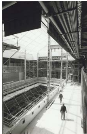
9 th Floor Renovations
