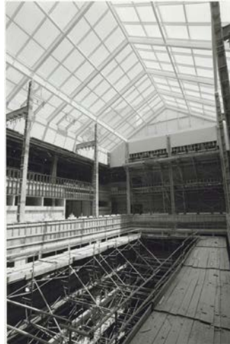
9 th Floor Renovations
