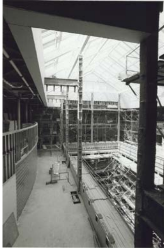
9 th Floor Renovations
