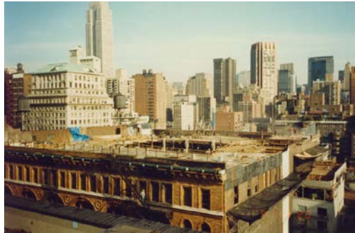
Scaffolding on the Roof After 1990 (From the Baruch College Archives)
