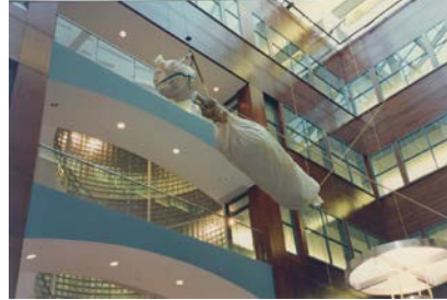
Library Renovation in Progress (From the Baruch College Archives)
